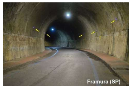
Fig. 1 Road tunnel test site (Framura – SP).
